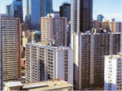
BREAKING THE BACKLOG
